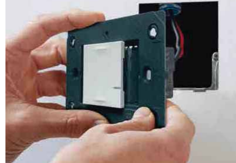
INSTALL NEW SMART DIMMER SWITCH ON WALL
